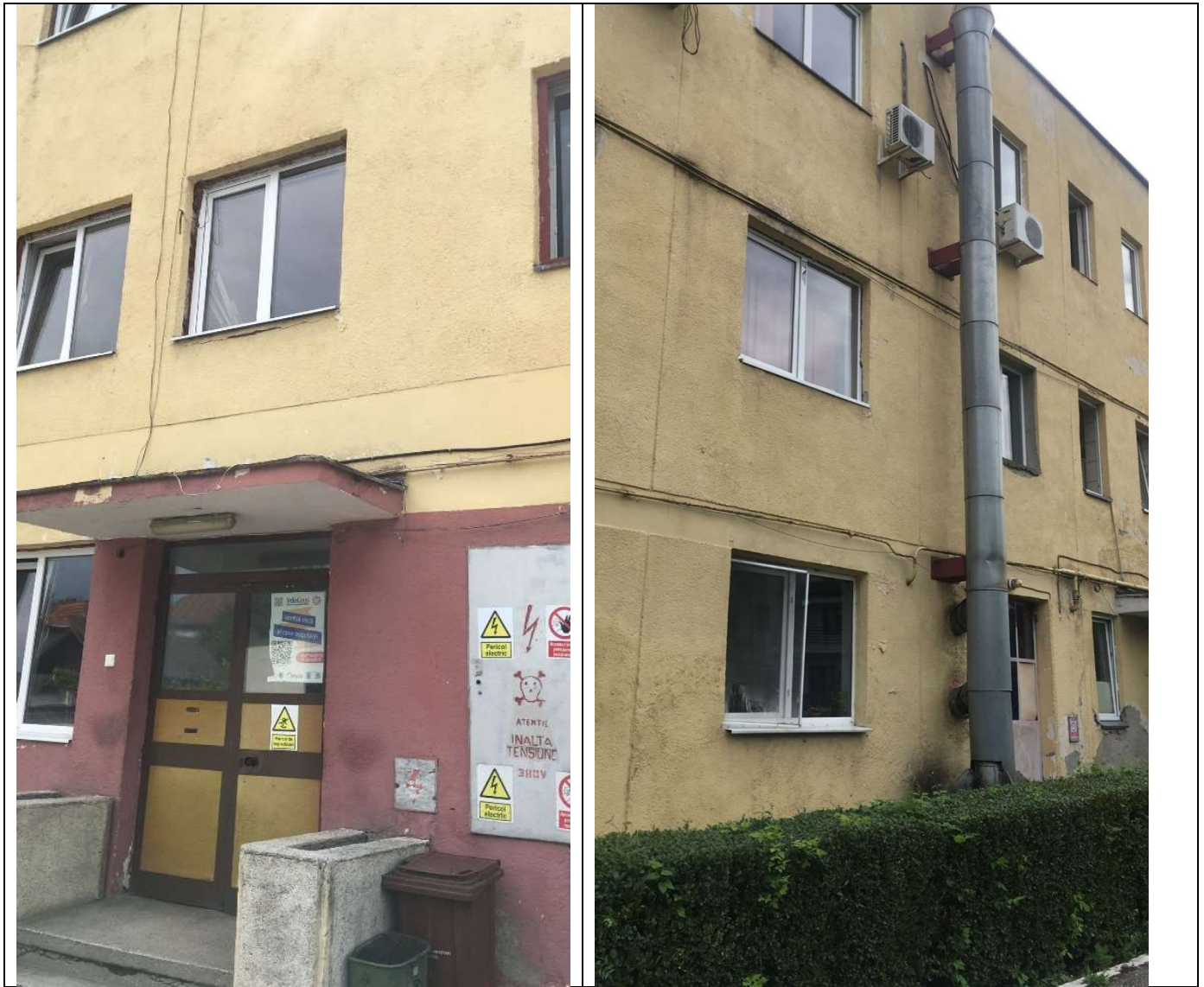
Fig 9 Existing AESI and PFD's C2 administrative building
